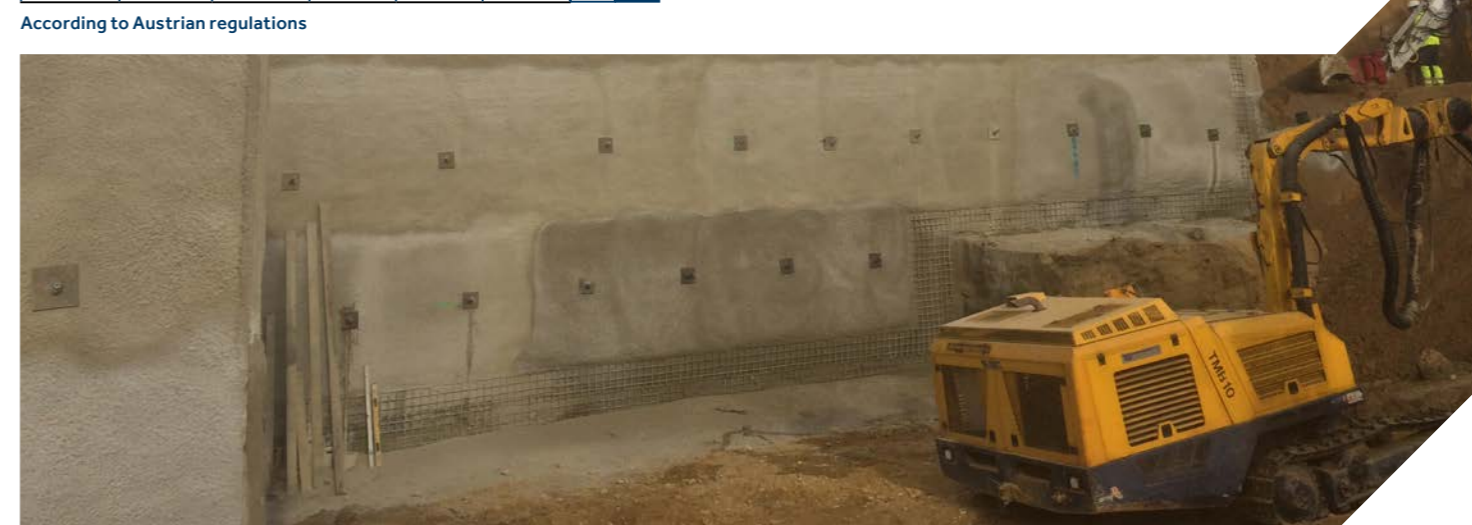
Soil nail with hollow bar
